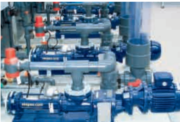
Pumps of range BN 2-6L Conveying product: Polymer solution Conveying capacity: 500–2500 l/h (2.2–11 GPM) • Pressure: 2 bar (30 psi) Temperature: 5–40 °C (41–104 °F)
