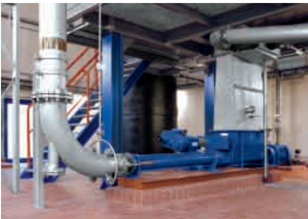
System solution with a BTI range pump with additional storage hopper and integrated level control, dry run protection (TSE) and boundary injection system
