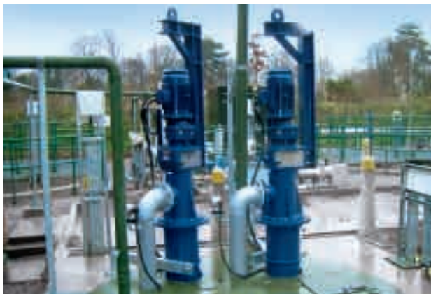
Pumps of range BE 70-12 Conveying product: Primary sludge Conveying capacity: 21 m 3 /h (92 GPM) • Pressure: 3 bar (45 psi) Temperature: 20 °C (68 °F)
