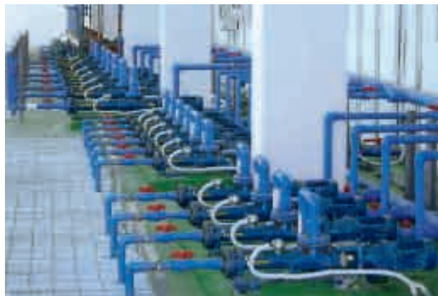
Pumps of range BN 5-6L Conveying product: Polymer solution Conveying capacity: 4500 l/h (20 GPM) • Pressure: 4.5 bar (67.5 psi) Temperature: 20 °C (68 °F)
