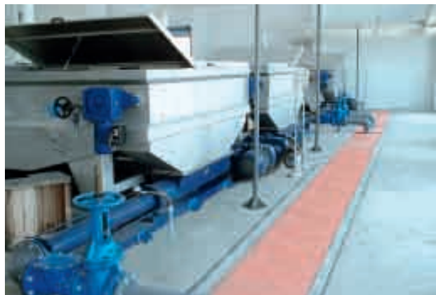
Pumps of range BT 35-24 Conveying product: thickened sludge Conveying capacity: 3–15 m 3 /h (13–66 GPM) • Pressure: 15 bar (225 psi) Temperature: 20 °C (68 °F)
