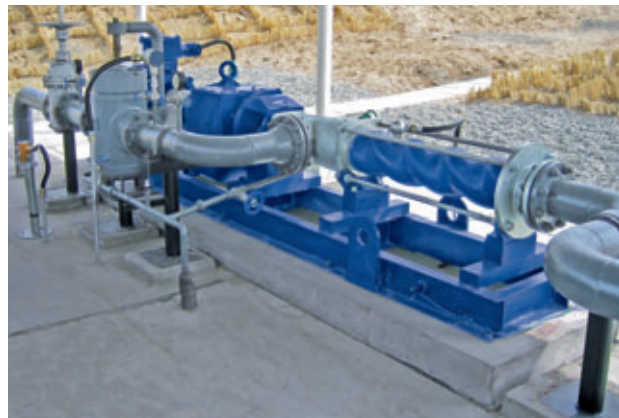
Pump of range BN 70-12V Conveying product: Crude oil Conveying capacity: 55 m 3 /h (242 GPM) • Pressure: 22 bar (319 PSI) Temperature: 10–50 °C (50–122 °F)
