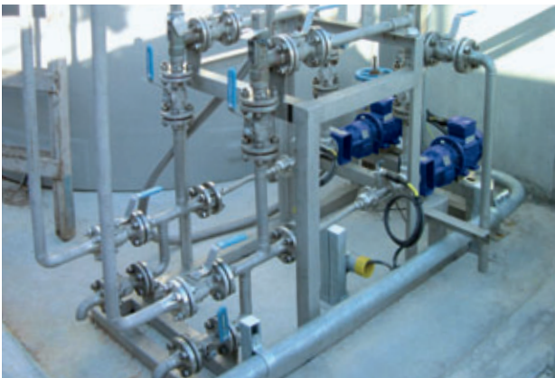
Pumps of range MD 012-12 Conveying product: Chemicals Conveying capacity: 33 l/h (0.145 GPM) • Pressure: 10 bar (145 PSI) Temperature: 60 °C (140 °F)
