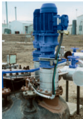
Pumps of range BE 70-12 and 35-6L Conveying product: Slop oil drains Conveying capacity: 48/17 m 3 /h (211/75 GPM) • Pressure: 8/6 bar (116/87 PSI) Temperature: 37 °C (98 °F)
