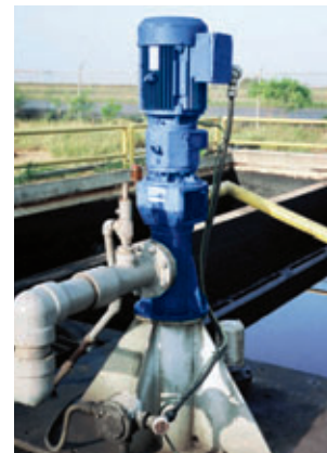
Pumps of range BE 70-12 and 35-6L Conveying product: Slop oil drains Conveying capacity: 48/17 m 3 /h (211/75 GPM) • Pressure: 8/6 bar (116/87 PSI) Temperature: 37 °C (98 °F)
