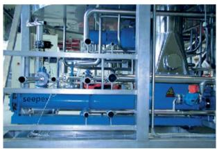
Pump of range BT 17-12 Conveying product: Draff Conveying capacity: 8 m³/h (35 GPM) Pressure: 4 bar (58 PSI) • Temperature: 80 °C (176 °F)
